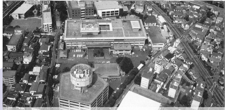
The Tokyo Plant before the shift to the Tsukuba Plant (around 1986)
